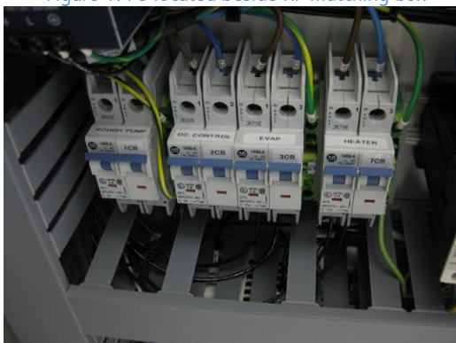
Figure 3: Breaker switches
